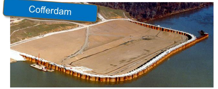
Concrete structure on permeable soils with "Sheet Pile "cut-off wall"
