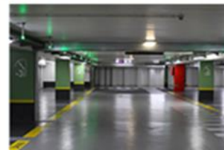
Underground car parks
