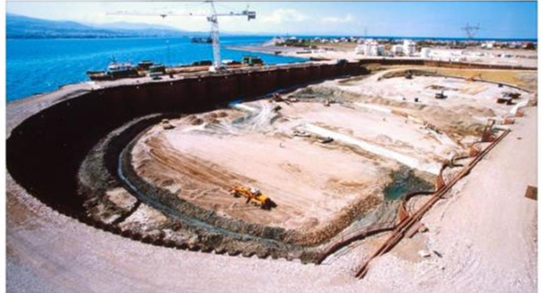
Sheet Pile cofferdam is removed to open dock and swim out concrete bridge column afloat.
