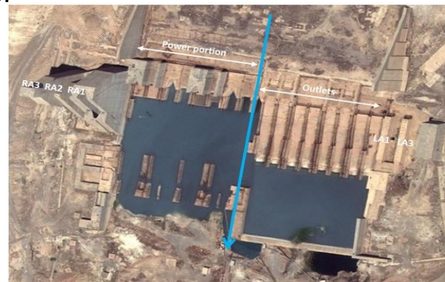
Current Situation of Badush Dam
