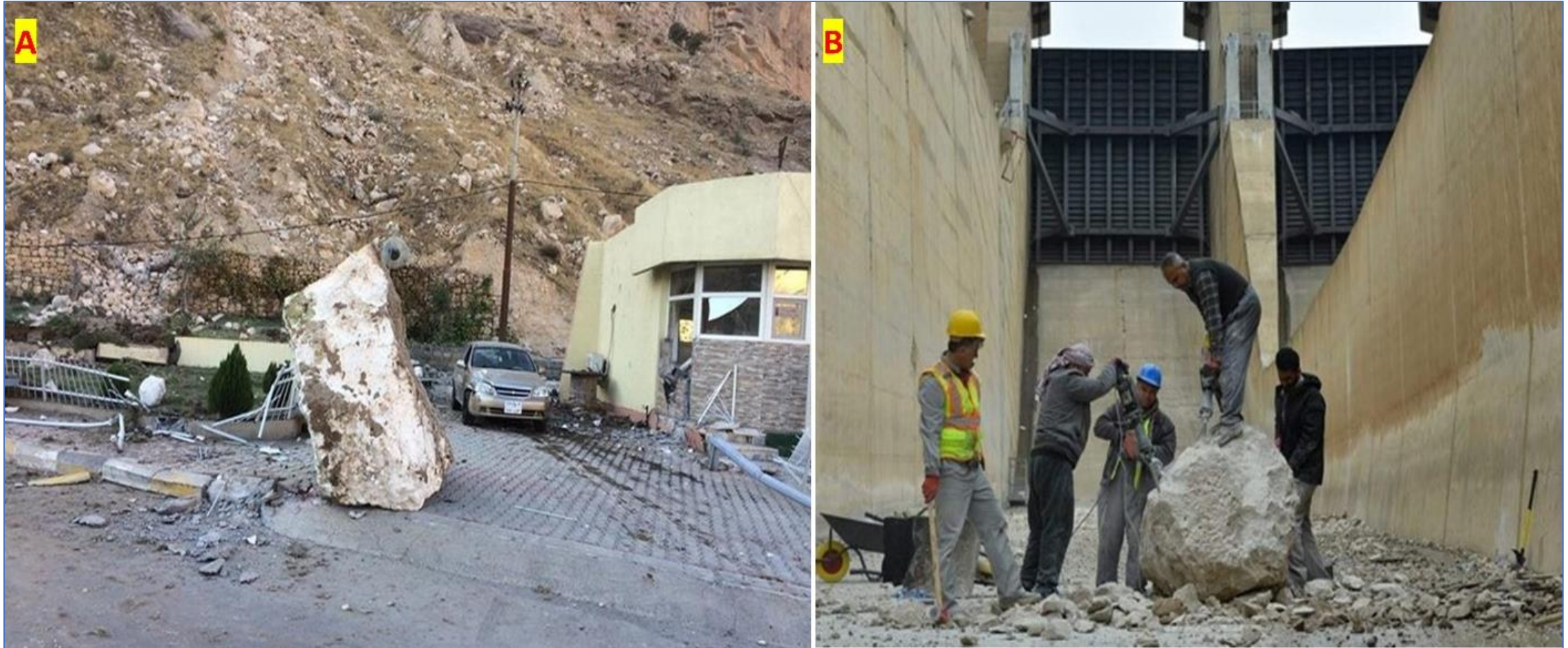
Figure 6: A- The Control Room, B- Pieces of Rock Fall at the Spillway Chute.
